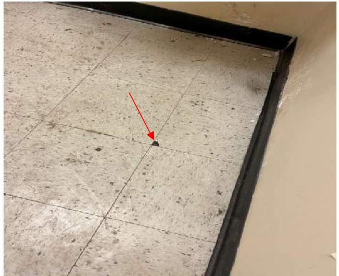
PHOTO No. 8 Typical View of ACBM Black Floor Tile Mastic
