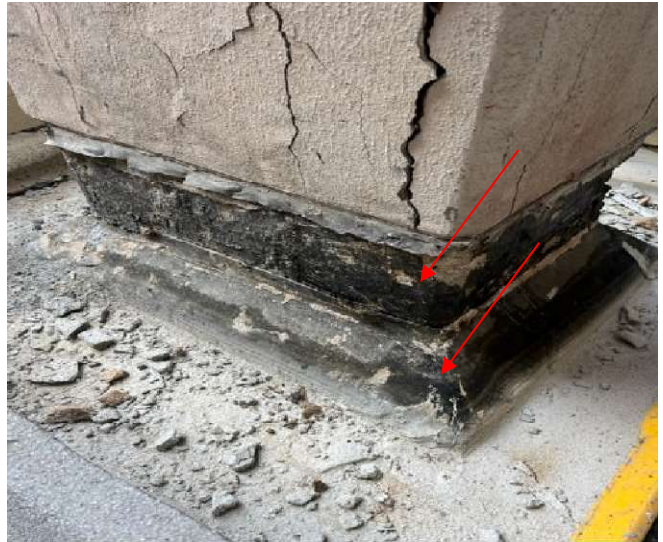
PHOTO No. 10 Typical View of ACBM Roof Flashing Sealant
