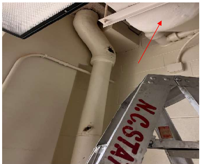
PHOTO No. 12 Typical View of Assumed ACBM Transite Pipe in Lab 113 next to ACBM Roof Drain Line
