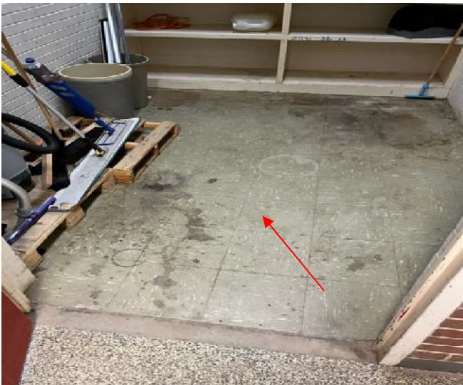
PHOTO No. 11 Typical View of ACBM 12" Green Floor Tile
