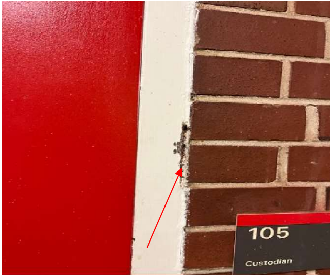
PHOTO No. 9 Typical View of ACBM Interior Door Caulking
