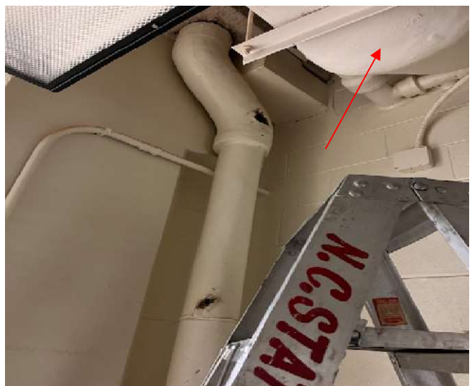
PHOTO No. 12 Typical View of Assumed ACBM Transite Pipe in Lab 113 next to ACBM Roof Drain Line
