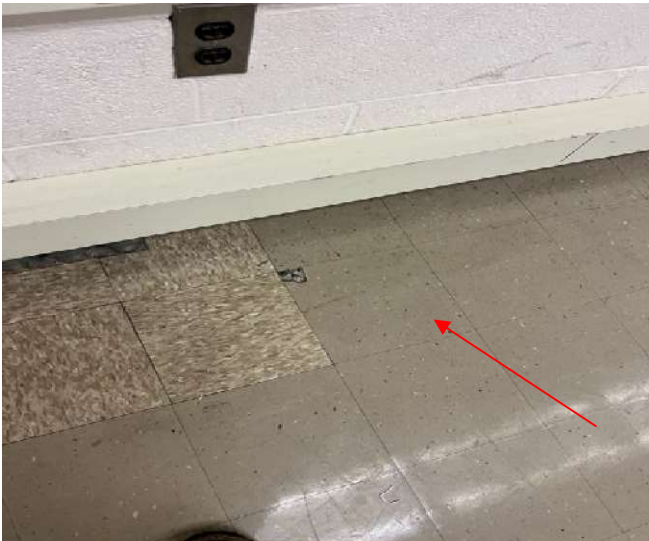
PHOTO No. 7 Typical View of ACBM 9" Gray/white Floor Tile & Black Mastic
