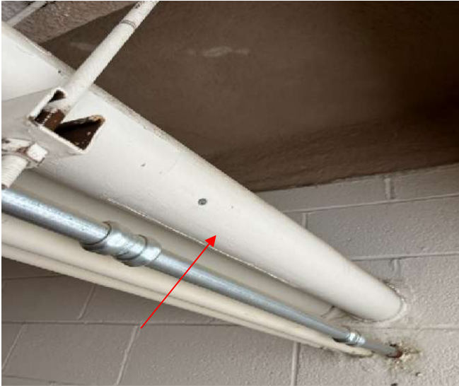
PHOTO No. 5 Typical View of ACBM 4" White Pipe Insulation
